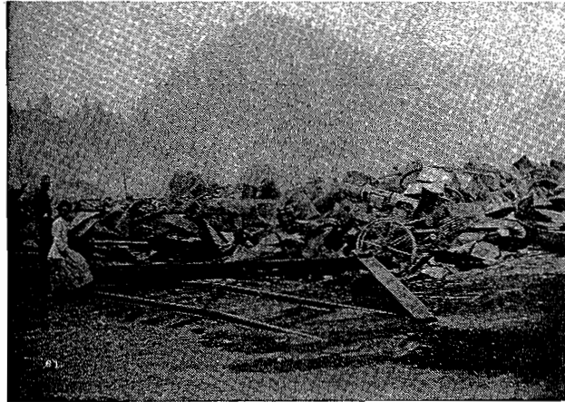
Coeur d' Alene Hardware Warehouse ruins after the August 20 fire. (Wallace, Idaho).
